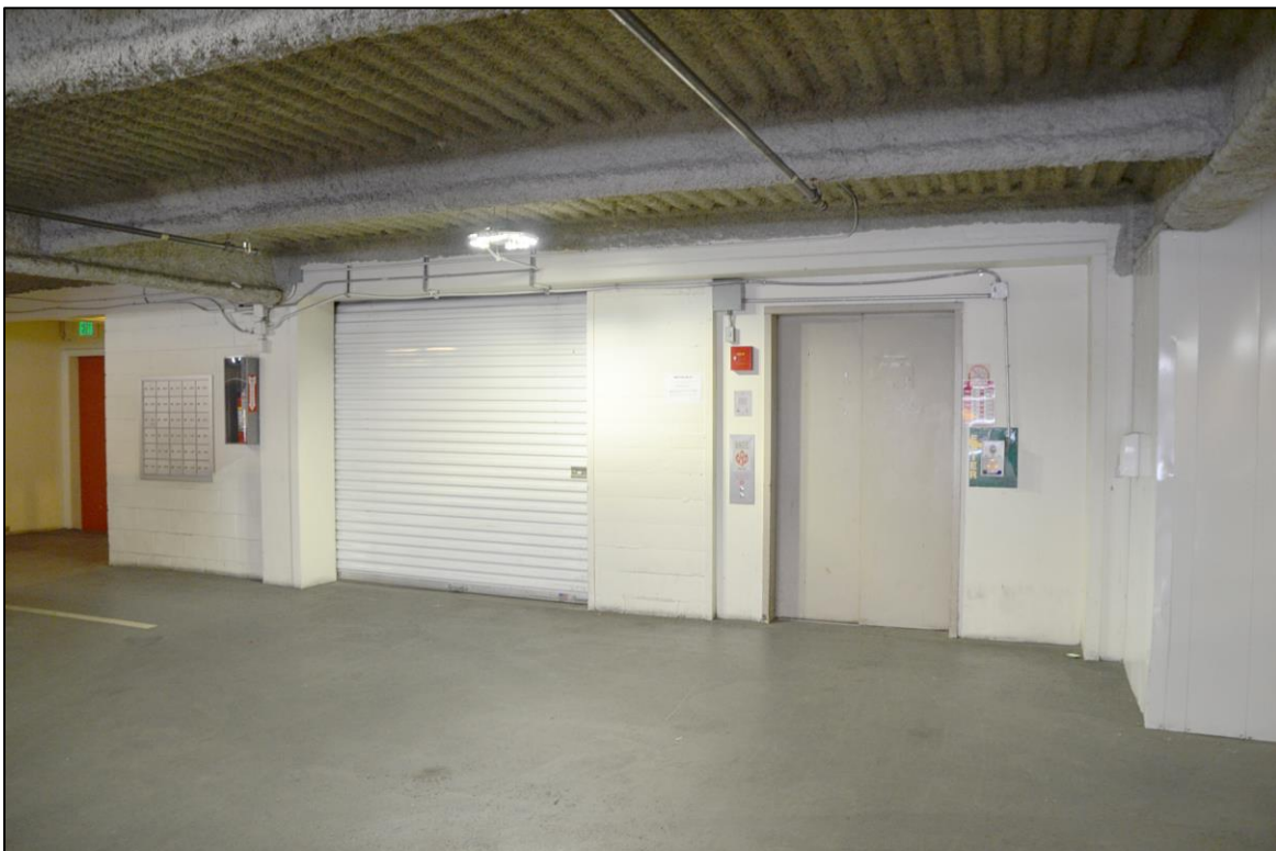
Figure 45. Freight elevator at former location of car elevators, ground level.
