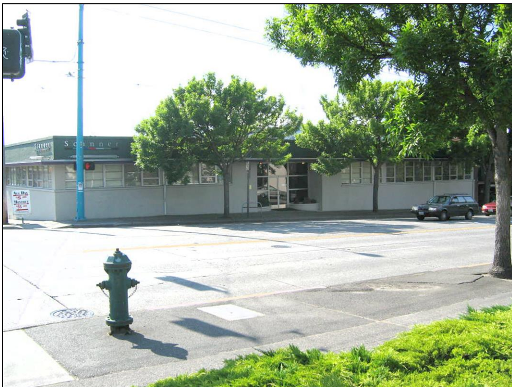
Figure 91. Addressograph Multigraph Agency Building (now demolished) (image courtesy of City of Seattle Department of Neighborhoods).
