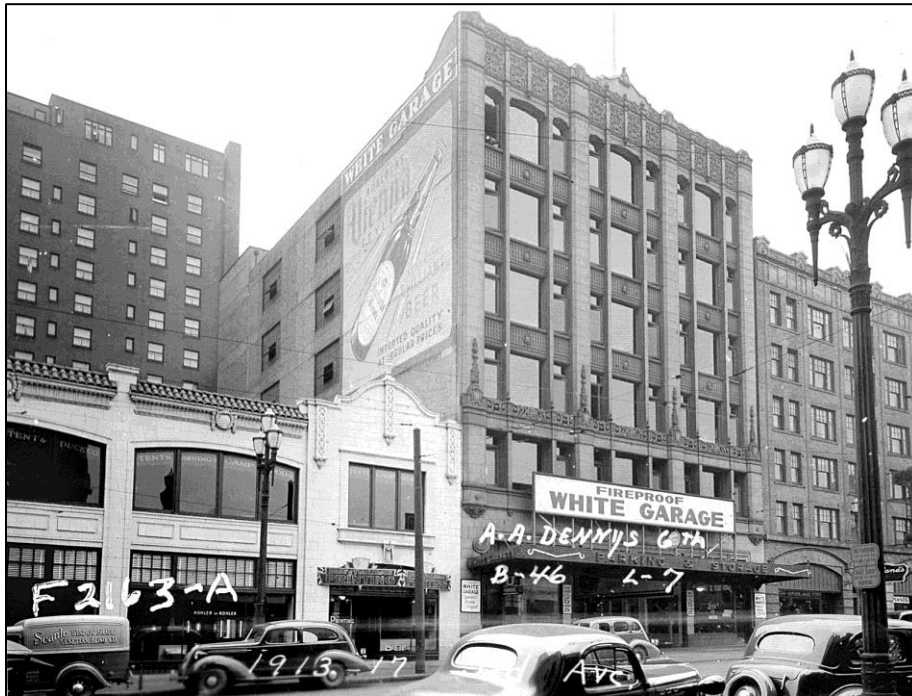
Figure 57. White Garage in 1930s. Note storefront windows to either side of garage entrance and canopy over sidewalk. Sign on the north and south ends of the building (at sidewalk level) advertise the convenience of the building and its fireproof construction. Note also the Chicago-style tripartite windows (King County Assessor 1938-1978).
