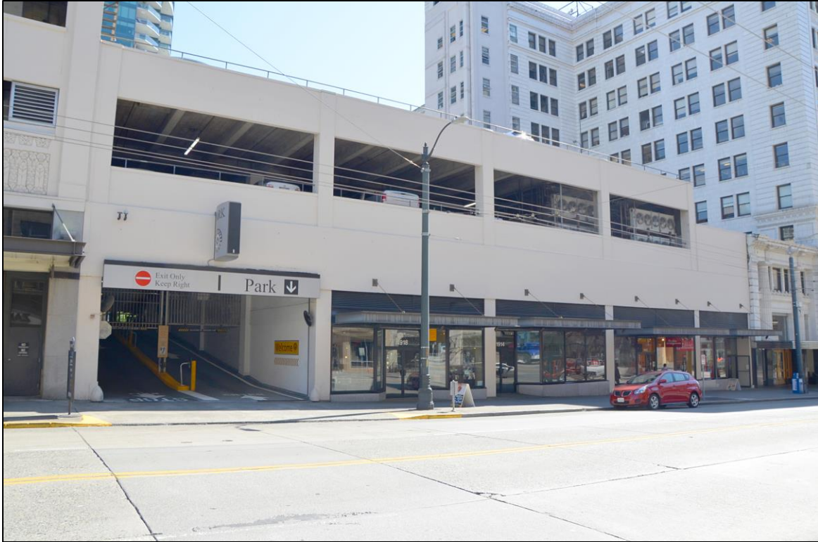
Figure 17. Securities Building Parking Garage.
