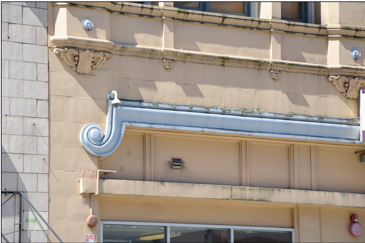
Figure 37. Detail of terra cotta above storefront.
