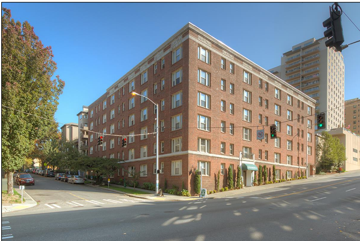
Figure 75. The Stockbridge Apartments (image courtesy of the Stockbridge Apartments).
