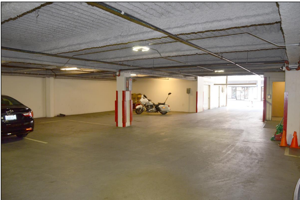
Figure 43. Ground level interior, view of parking area and garage entrance.
