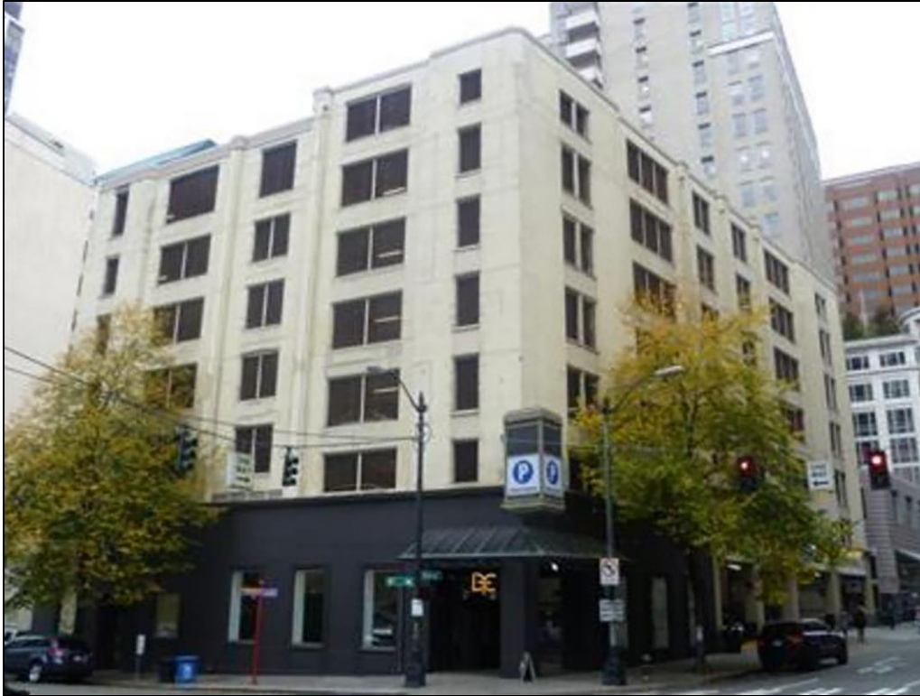
Figure 66. Fox Garage, following removal of parapet and exterior ornamentation in 2012 (image courtesy of King County Department of Assessments).
