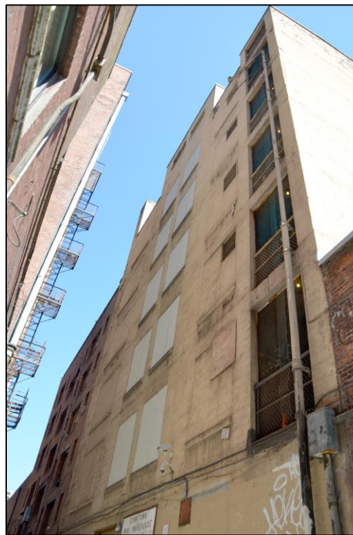
Figure 27. Rear (west) elevation of building, viewed from the alley between 2nd and 3rd Avenues.
