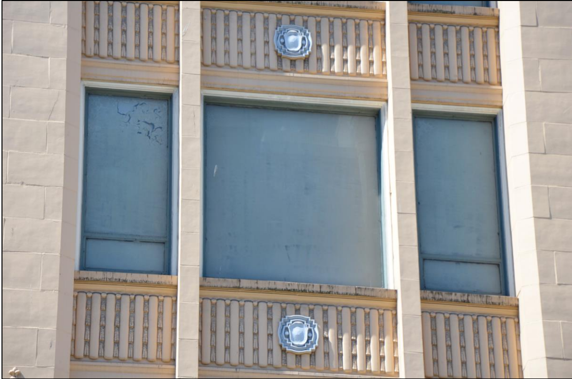
Figure 38. Detail of terra cotta and windows on 4th floor.
