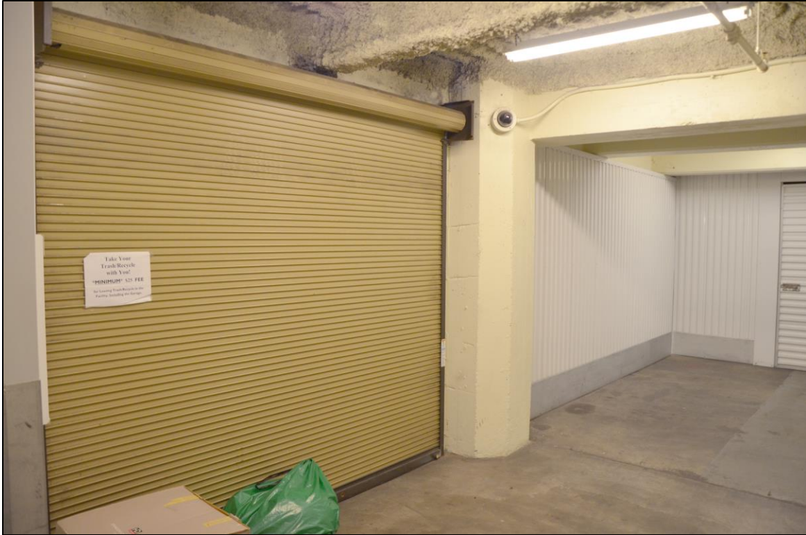
Figure 48. Loading bay on Mezzanine level (west side of building).
