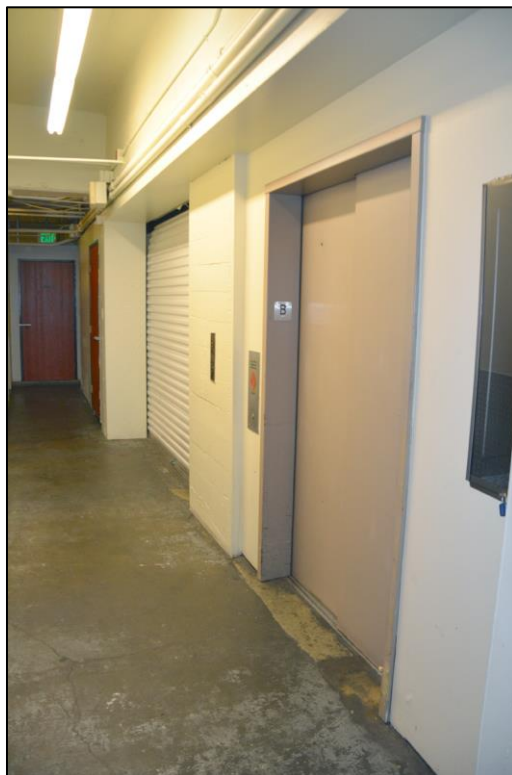
Figure 53. Freight elevator at former location of car elevators.
