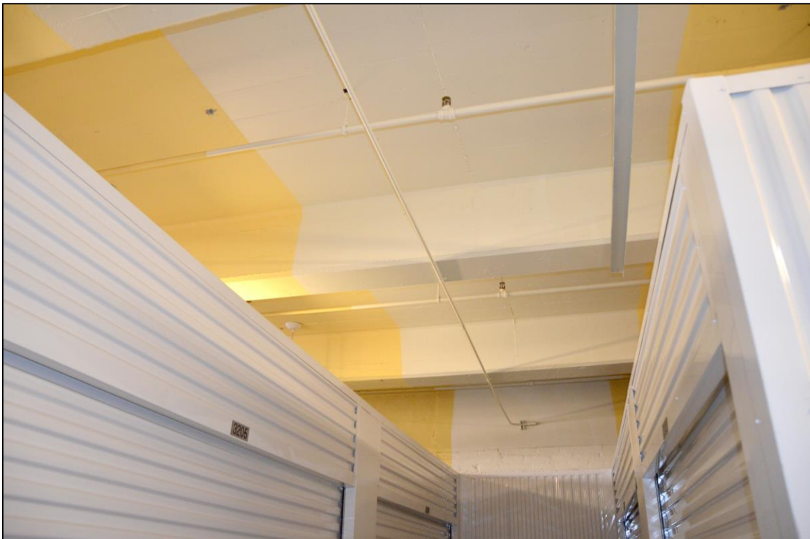
Figure 51. Reinforced concrete construction visible above storage units.
