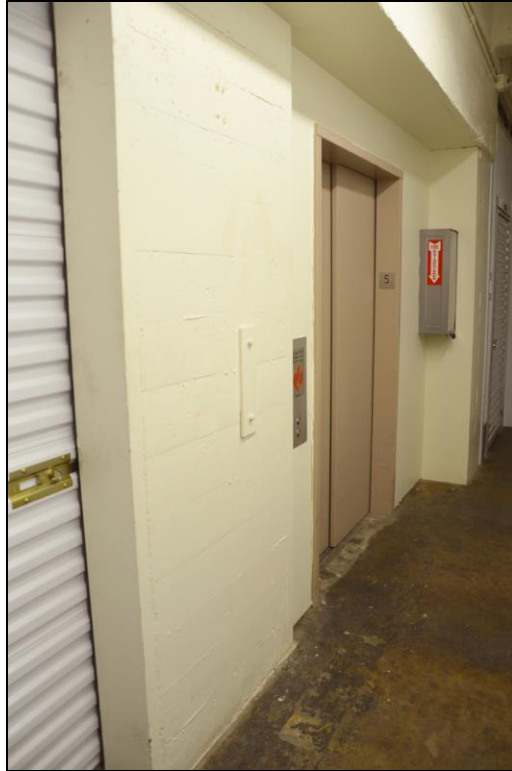
Figure 52. Former location of car elevators.
