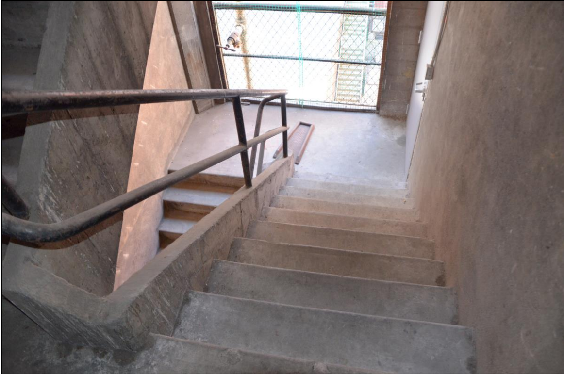
Figure 54. Stairwell at southwest corner of building, showing opening in exterior wall.
