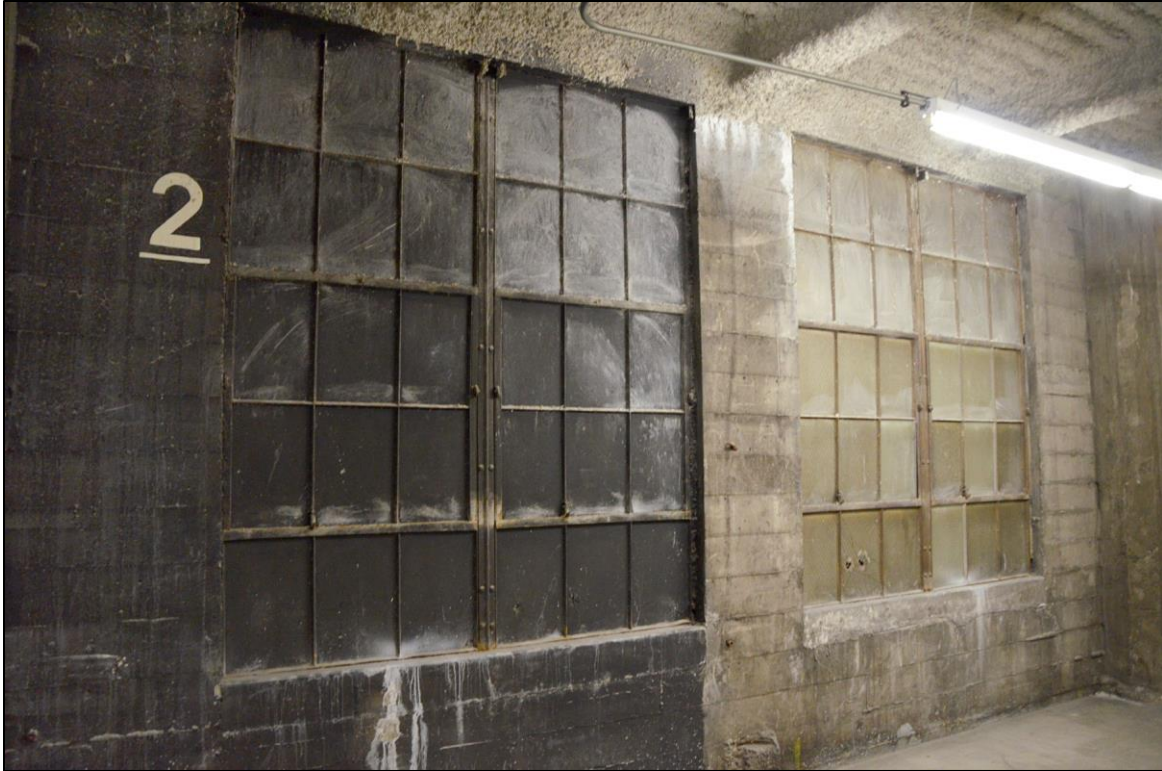
Figure 42. Steel sash on west (alley) façade, viewed from interior.
