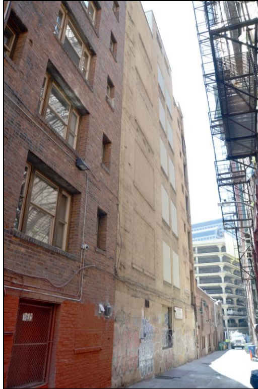
Figure 30. West elevation, view to south.
