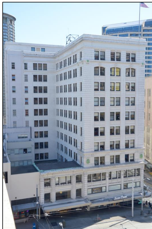
Figure 16. Securities Building, viewed from roof of White Garage.
