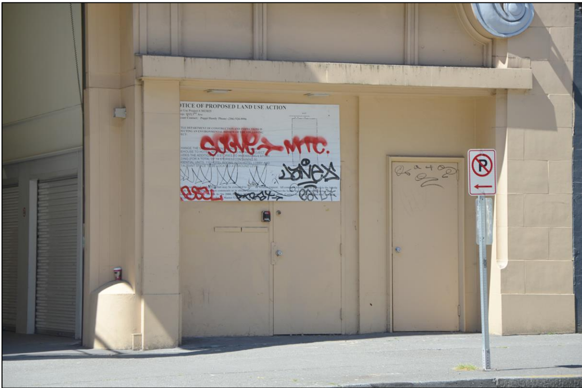
Figure 41. Stairway door at northeast corner of building.
