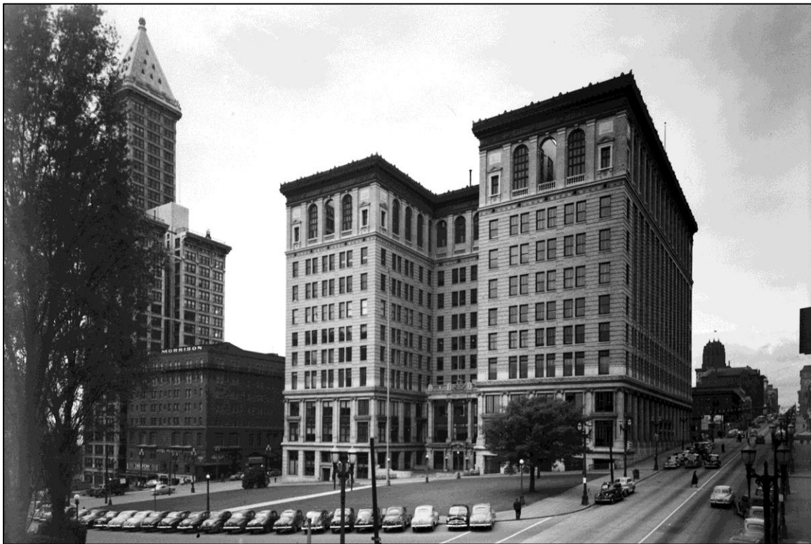
Figure 69. King County Courthouse in 1949, showing the addition designed by Bittman in 1931 (Image No. 9347, Seattle Municipal Archives).
