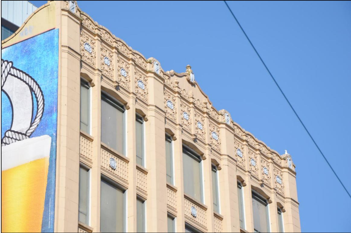
Figure 34. Detail of terra cotta above sixth floor.
