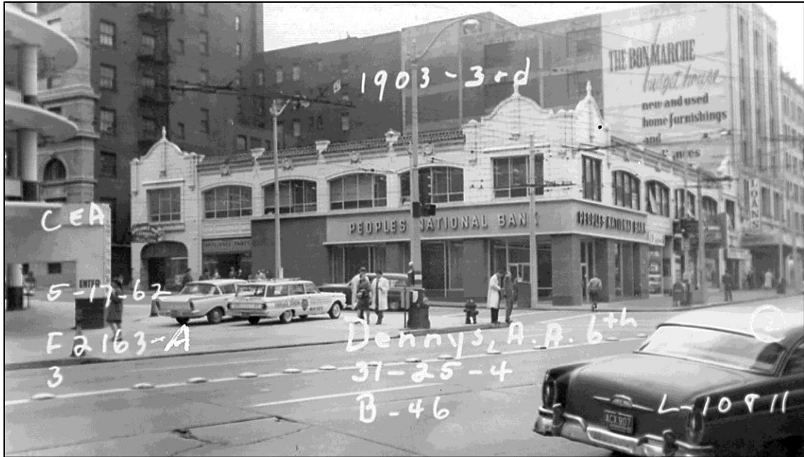
Figure 61. 1962 image showing 1915 3rd Avenue as the Bon Marche Budget House (note advertisement on south side of building) (King County Assessor 1938-1978).
