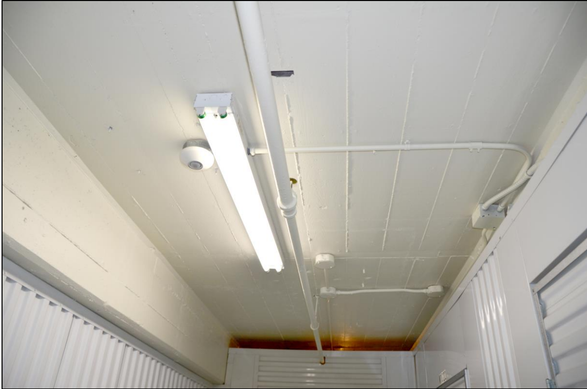
Figure 46. Reinforced concrete construction is visible in some areas between storage units.
