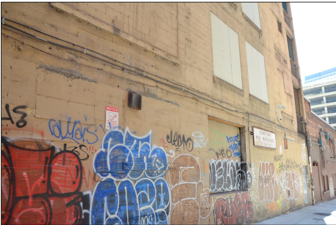
Figure 29. Loading door and exterior of mezzanine level, viewed from alley.
