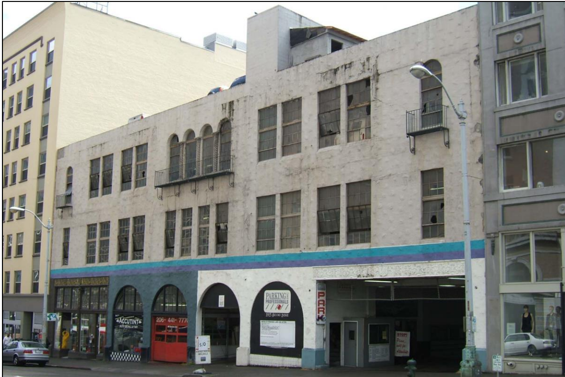
Figure 67. Northwest Building Company Garage, demolished in 2012 (image courtesy of the City of Seattle Department of Neighborhoods).
