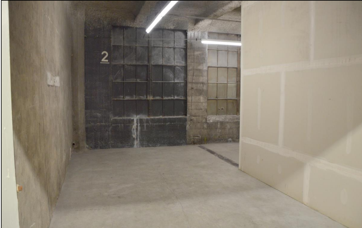
Figure 50. Interior of storage unit on west side of building, showing steel sash that are covered on the exterior.
