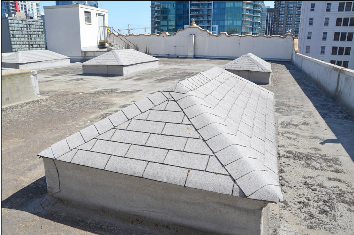
Figure 32. Covered skylights on roof; view to northeast.
