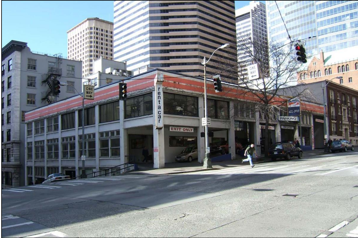
Figure 64. Campbell Building Garage (image courtesy of the City of Seattle Department of Neighborhoods).
