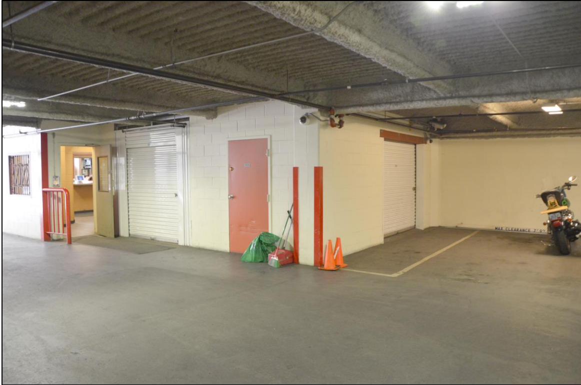
Figure 44. Office area on ground level, southeast corner of building.
