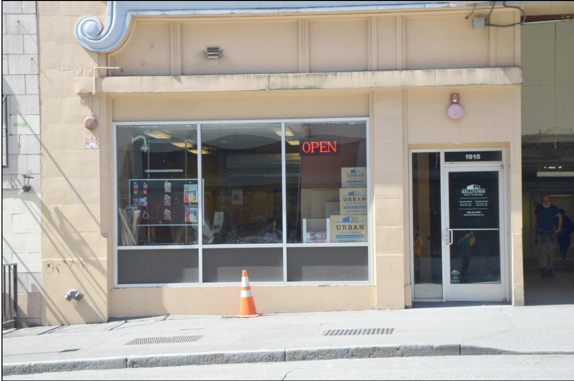
Figure 40. Storefront/office at southeast corner of building.
