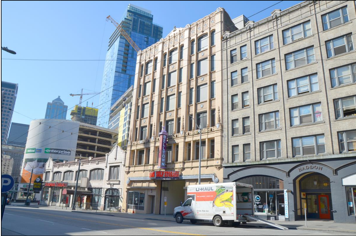
Figure 26. 1915 3rd Avenue, view south.
