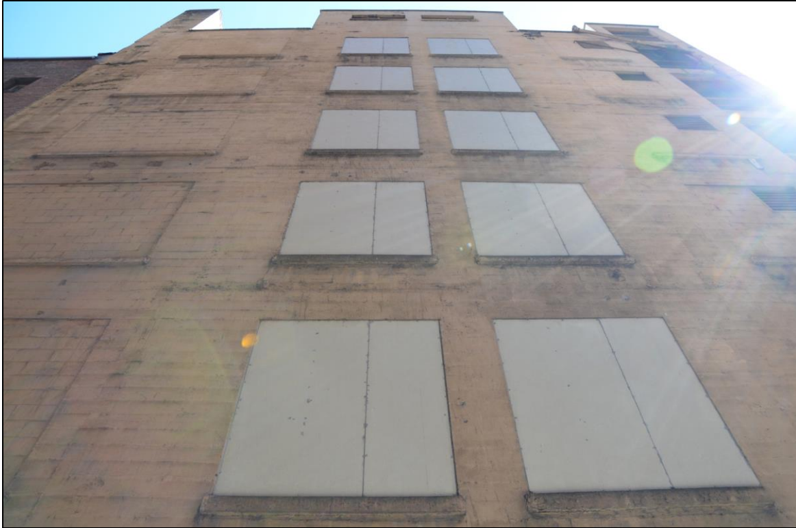
Figure 28. Infilled and covered windows on alley elevation.
