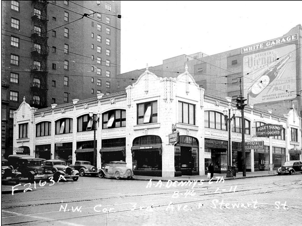
Figure 59. 1930s image showing south elevation of White Garage behind the Donohoe Garage (seen here as Doner Piano, Postal Telegraph and Puget Sound Tent and Duck Co.). Note steel sash next to beer advertisement: these have been removed and the openings have been infilled (King County Assessor 1938-1978).
