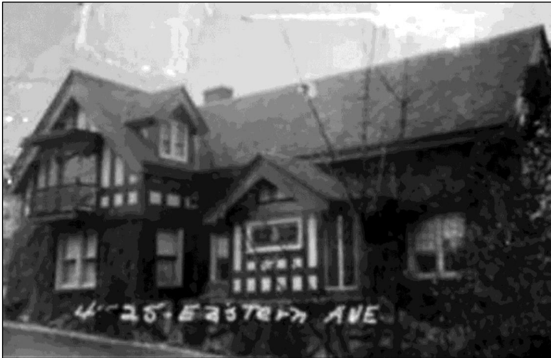
Figure 68. Bittman House (image courtesy of King County Department of Assessments).
