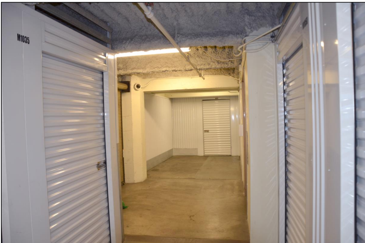
Figure 47. Typical view of interior, showing storage units.
