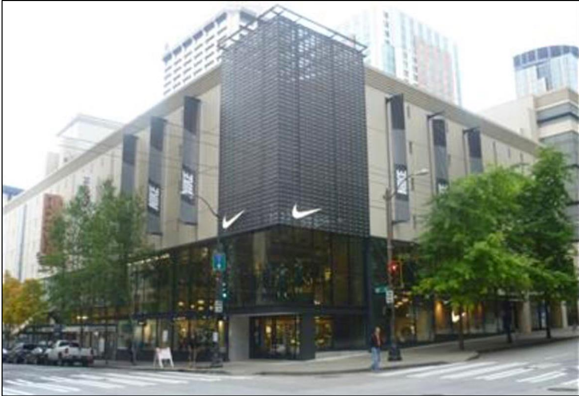
Figure 86. Ernst Hardware headquarters building after several major alterations (image courtesy of King County Department of Assessments).
