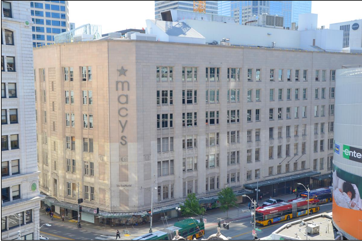
Figure 23. Bon Marche, viewed from roof of White Garage.
