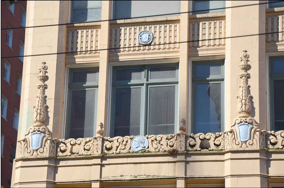
Figure 36. Detail of terra cotta and windows at third floor.
